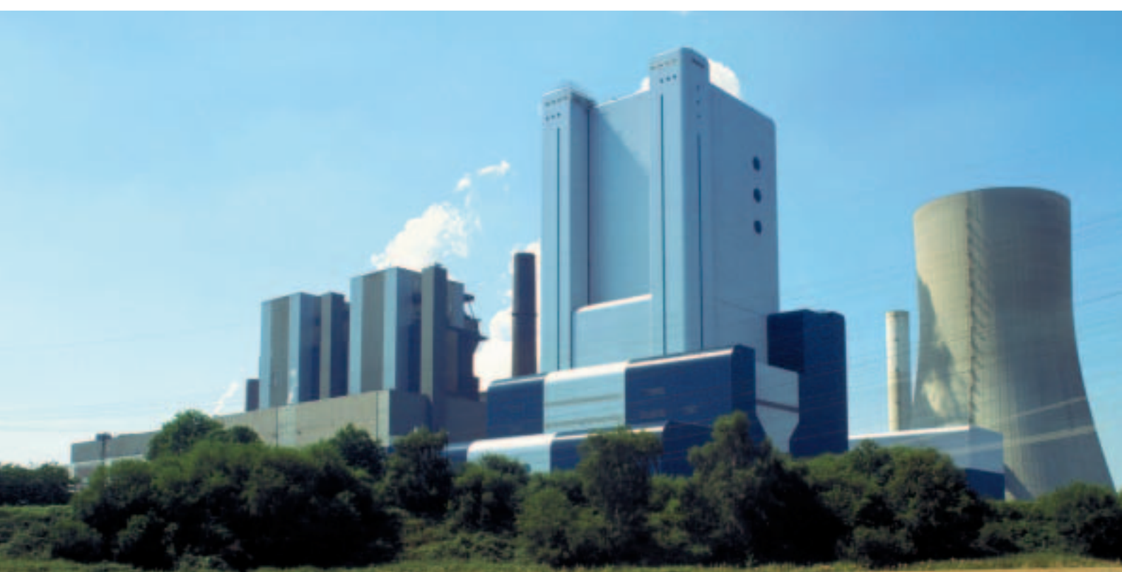
[Courtesy of Alstom Power]
